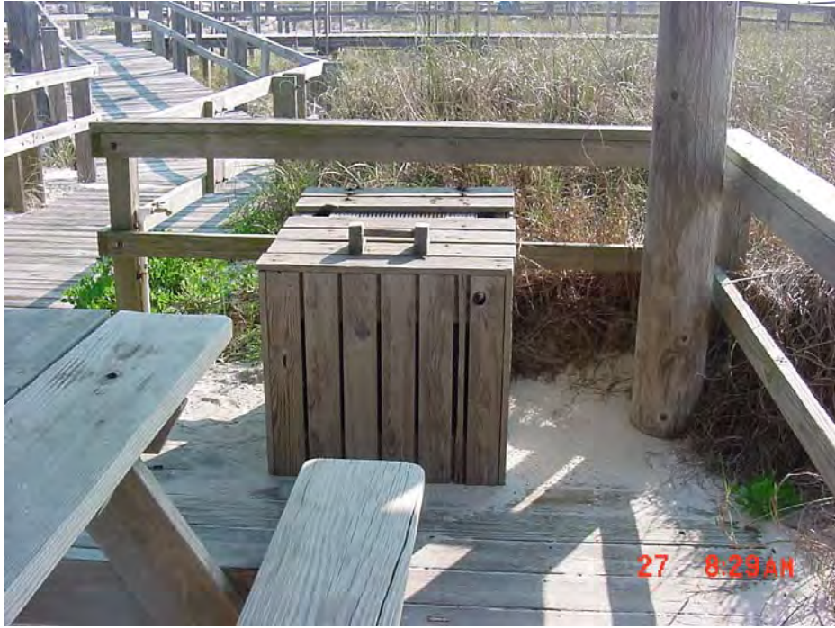
Example of trash receptacle that is secured and heavy enough not to easily be turned over.
