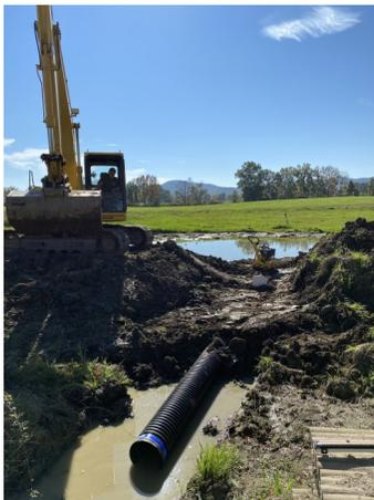
Conte staff installed a culvert and water valve in the newly created wetland at Fort River Division. We are hopeful that rain and snowmelt will refill the pond for an active spring season.
