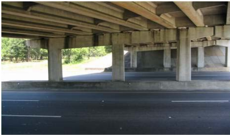
Photo 9: Staining on sides of pier caps
