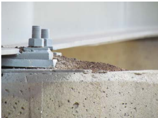
Photo 5: Guano deposit on pier, obscuring structural features.
