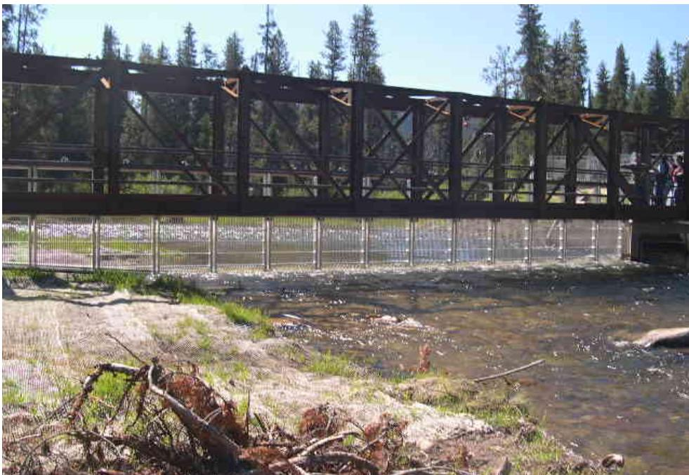
**Figure 2.** Bridge style weir like the one proposed for the Imnaha Facility.
