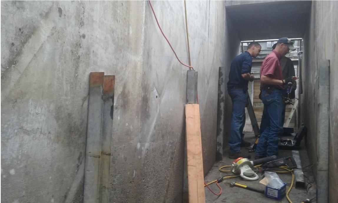
Figure 5. CTUIR Operations and Maintenance crews working on getting the lower Lookingglass trap working (May 2018). The first day consisted of drilling holes for the stations, boards were placed the following day.
