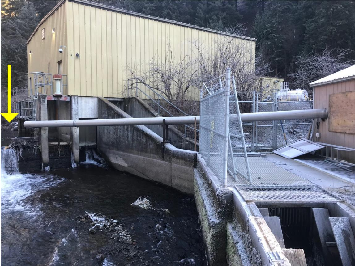
Figure 4. Lookingglass Hatchery return tube constructed by ODFW and CTUIR which allows fish to be released directly into the stream after handling. Pipe has running water, a gradual slope, and releases fish into a deep pool (arrow).
