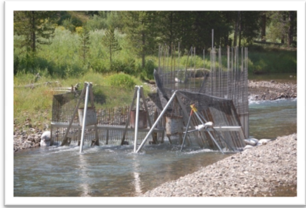
Figure 7. Five Mile Weir.
