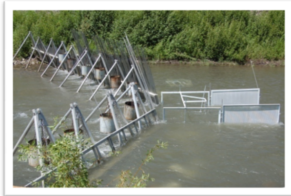
Figure 5. Final modification to Pole Flat Weir and Trap Box.
