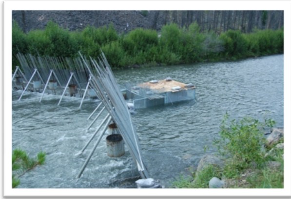
Figure 6. Pole Flat Weir and trap box.
