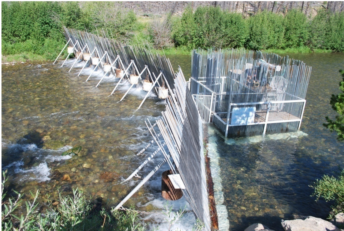
Figure 3. Pole Flat Weir and Trap Box.
