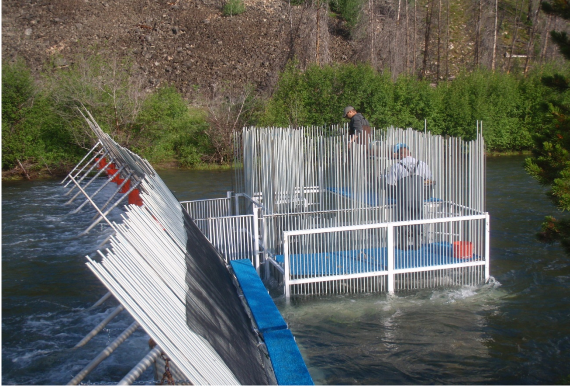
Figure 4. Pole Flat weir.
