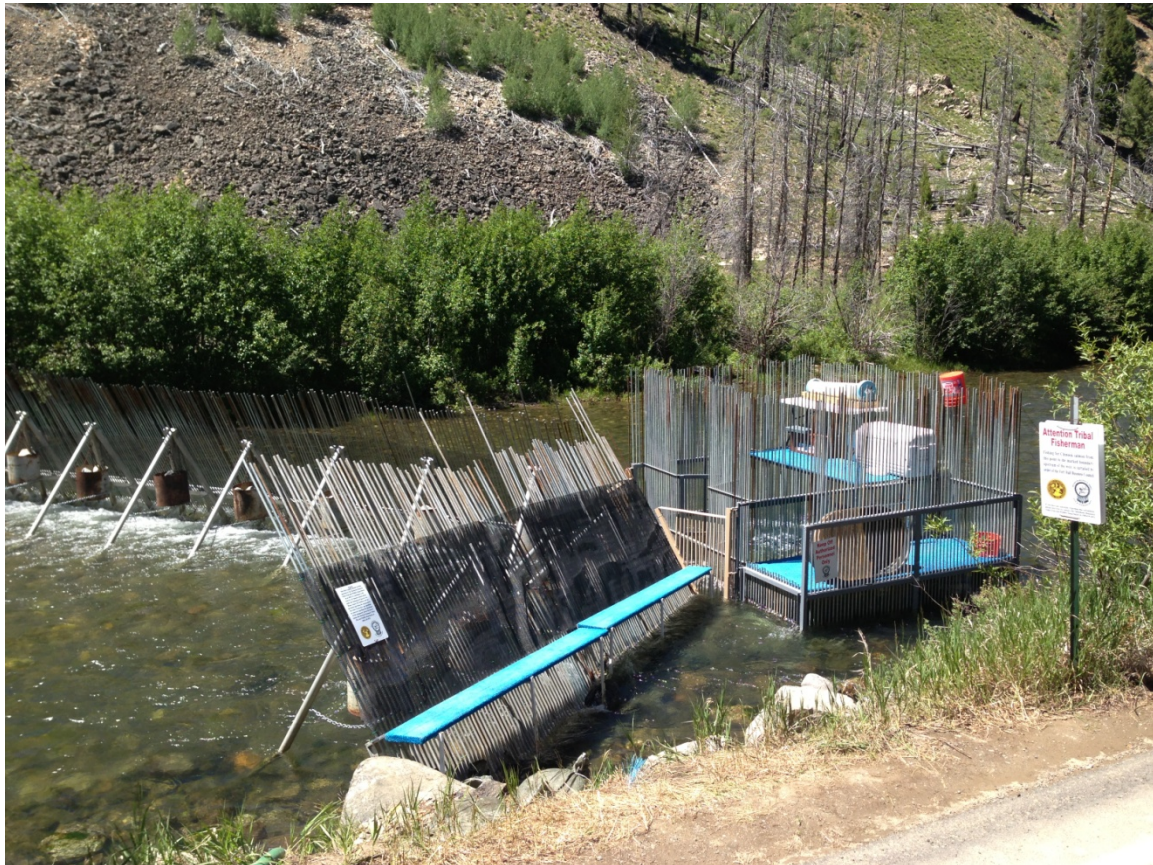
Figure 9. Pole Flat weir, catwalk, fish trap, live-wells, and work station.
