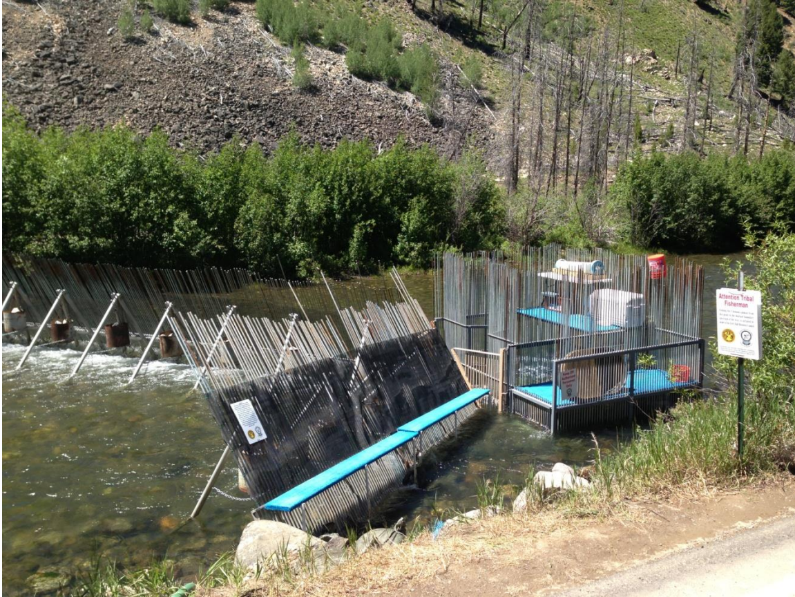
Figure 8. Pole Flat weir, catwalk, fish trap, live-wells, and work station.
