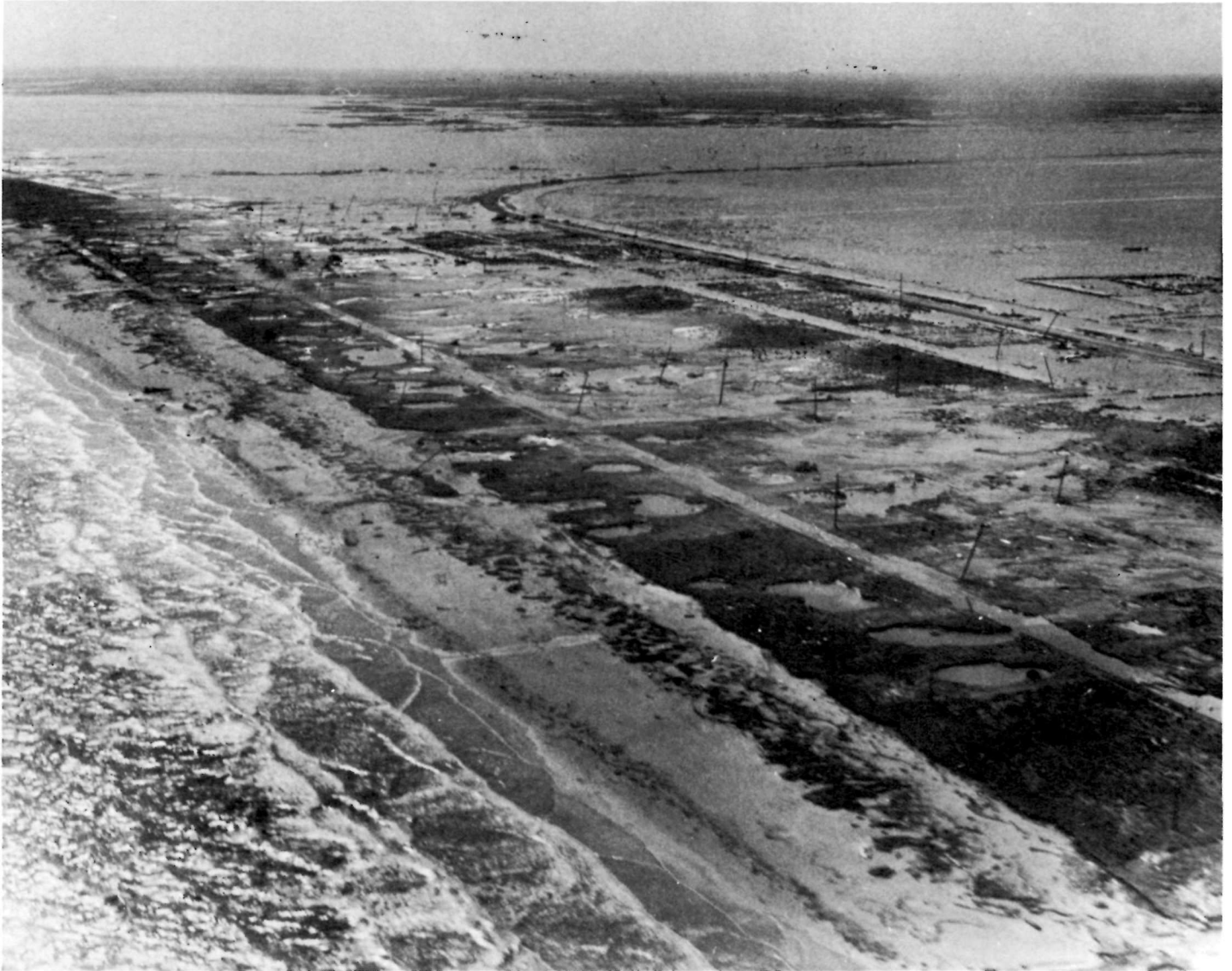
Damage to Holly Beach, LA, from Hurricane Audrey Bill Goffert
