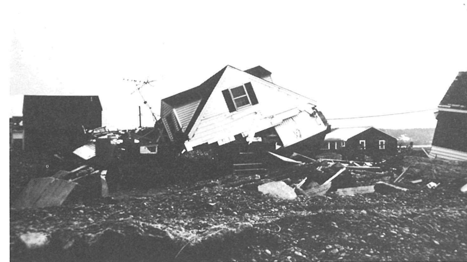
Scituate Beach, MA, after a storm, 1978 Sterling Wall
