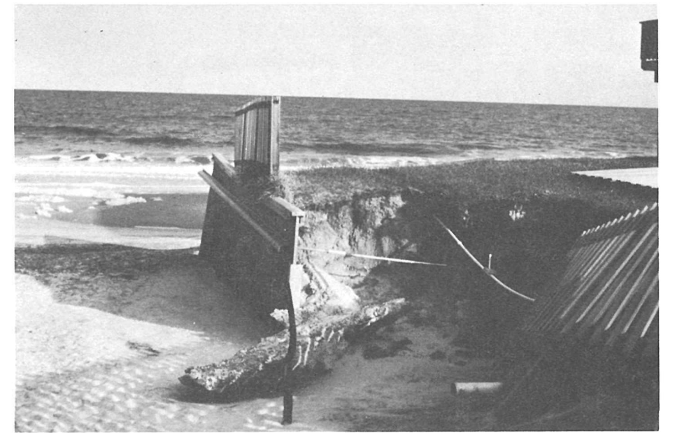
Falling seawall, Bethany Beach, DE Jim McFarland
