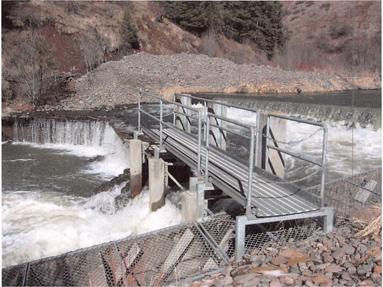
Figure 2. Lookingglass Hatchery adult fish trap located at rkm 4.0 on Lookingglass Creek near the hatchery water intake.
