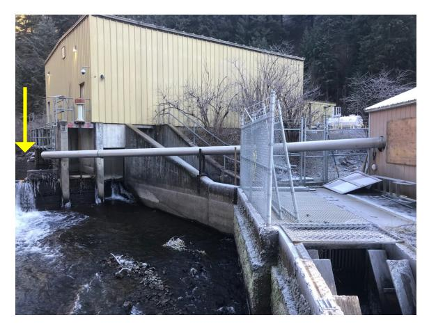
Figure 4. Lookingglass Hatchery return tube constructed by ODFW and CTUIR which allows fish to be released directly into the stream after handling. Pipe has running water, a gradual slope, and releases fish into a deep pool (arrow).
