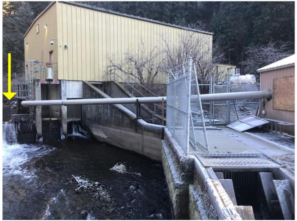
Figure 6. Lookingglass Hatchery return tube constructed by ODFW and CTUIR which will allow fish to be released directly into the stream after handling. The tube is still in need of a water pump to be fully functional. The arrow indicates the deep pool where passed adults were released.
