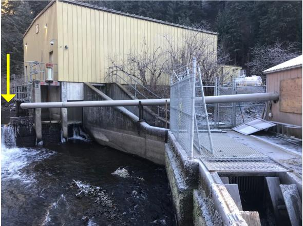
Figure 6. Lookingglass Hatchery return tube constructed by ODFW and CTUIR which will allow fish to be released directly into the stream after handling. The arrow indicates the deep pool where passed adults were released.
