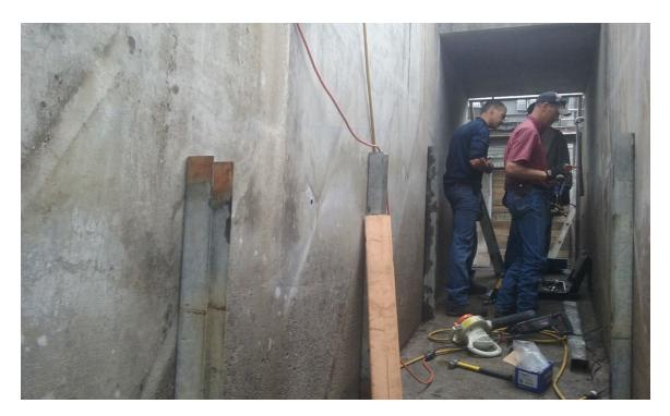
Figure 5. CTUIR Operations and Maintenance crews working on getting the lower Lookingglass trap working (May 2018). The first day consisted of drilling holes for the stations, boards were placed the following day.
