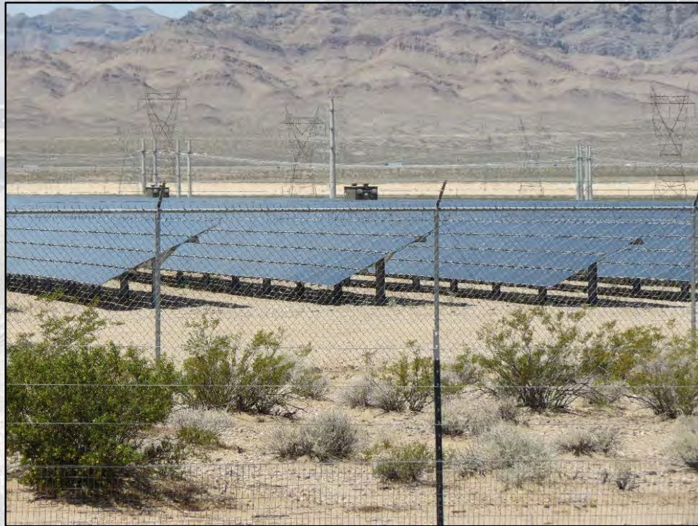
Graded and total removal
