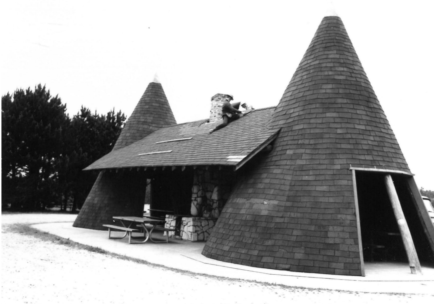
Photo 4: The Show Pool Shelter in the 1960s. The shelter appears to have lost its window openings.
