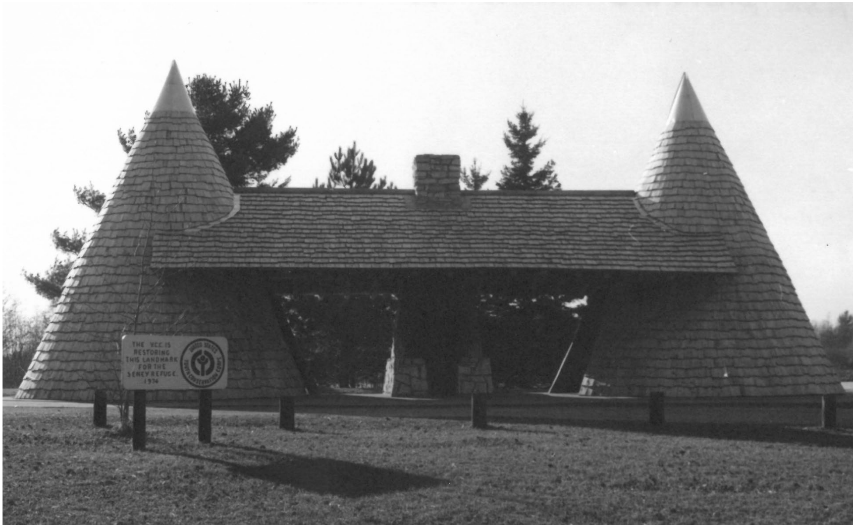
Photo 6: The Show Pool Shelter in 1974 after the work was completed.
