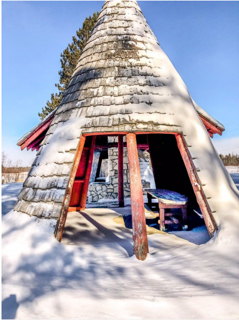
Photo 9. looking through doorways of structure in 2022.
