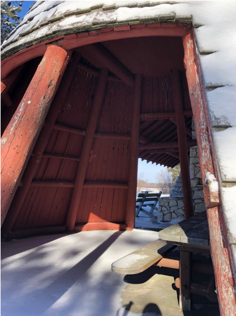
Photo 10. Interior View of Shelter in 2022.
