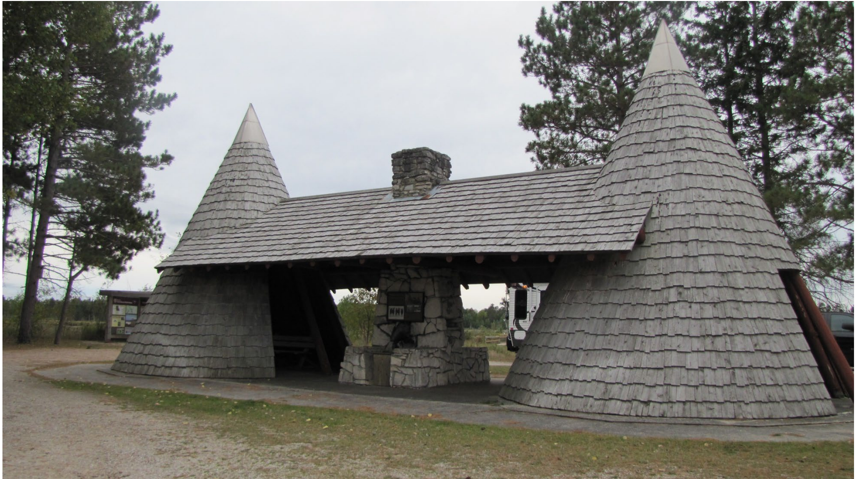
Photo 7: Current Structure as seen in 2015.
