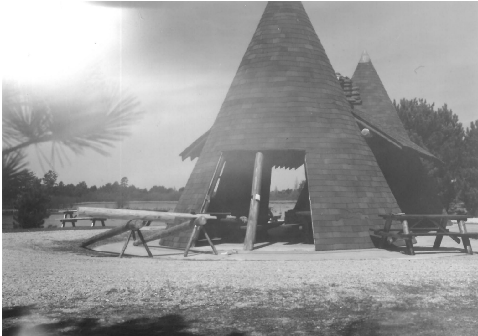
Photo 3: The Show Pool Shelter in 1955. The end doors have been added. It is now covered in asphalt shingles.
