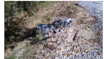
Ole Mill post-construction. Photo by USFWS
