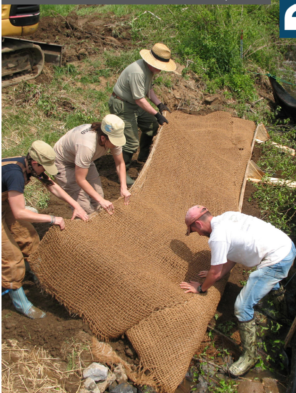
Streambank stabilization in North Carolina. Photo by USFWS
