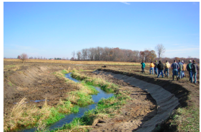
TWO-STAGE DITCHES CAN CAN REDUCE FLOODING UPSTREAM
