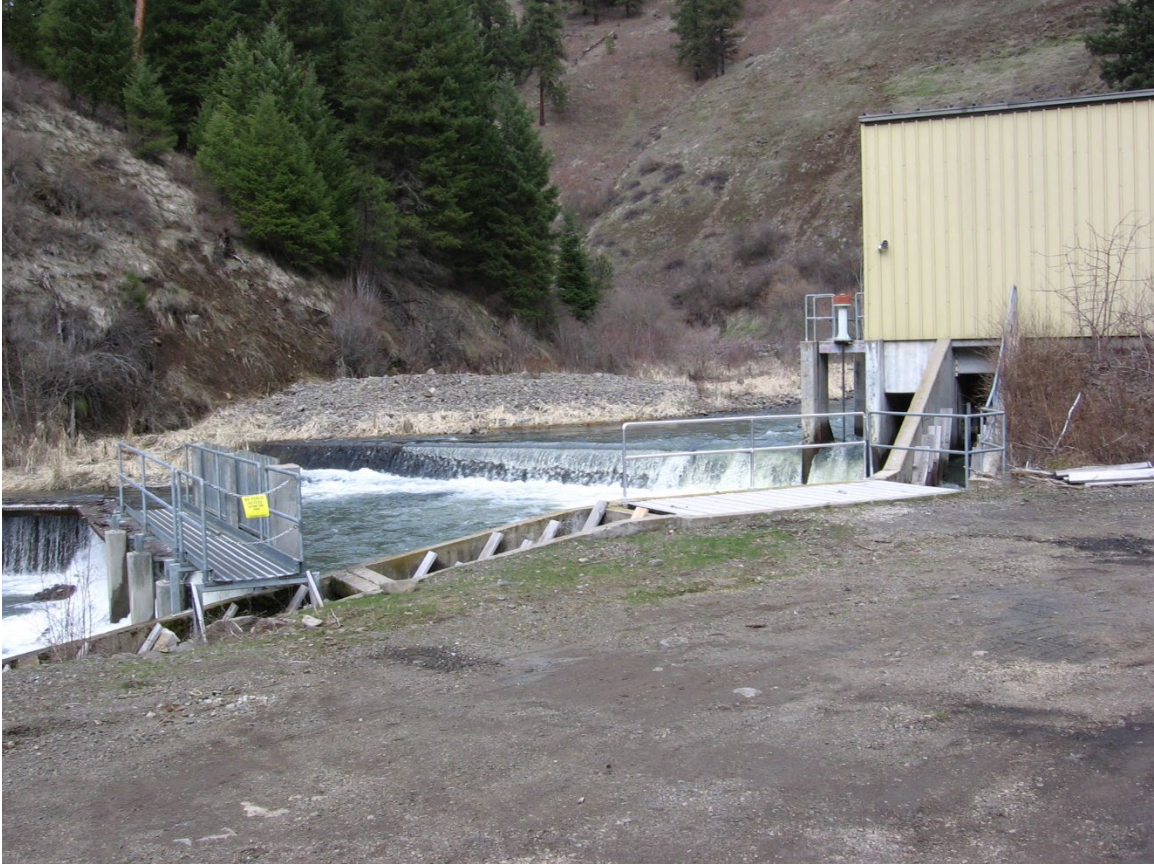
Figure 6. Lookingglass Hatchery upstream adult weir and ladder. Adults are released 0.4km upriver.
