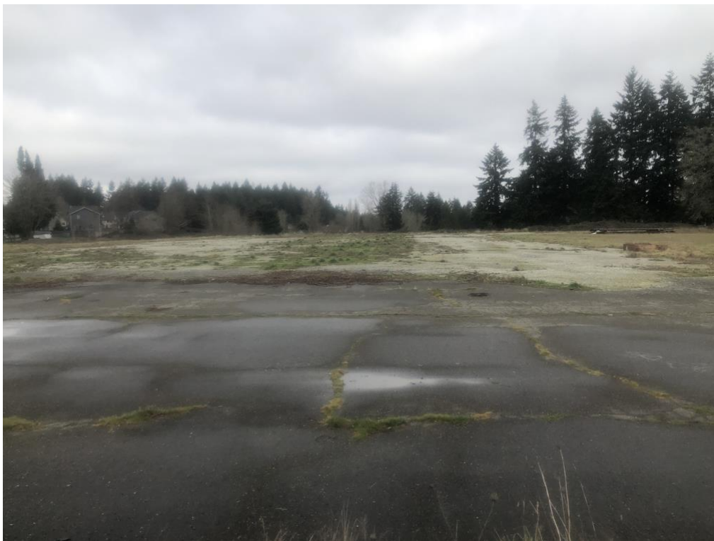
Photo 6. View north from PP3 of pavement and arena demolition site (January 15, 2021).
