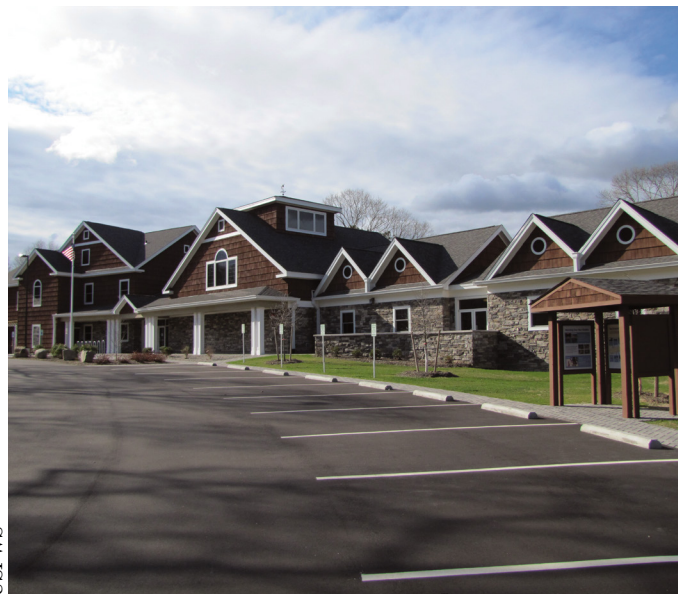
Long Island NWRC Visitor Center
