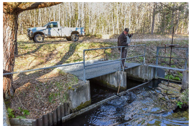
STAFF MEMBER AT PENDILLS CREEK NATIONAL FISH HATCHERY CLEANING THE WATER INTAKE. PHOTO COURTESY USFWS.
