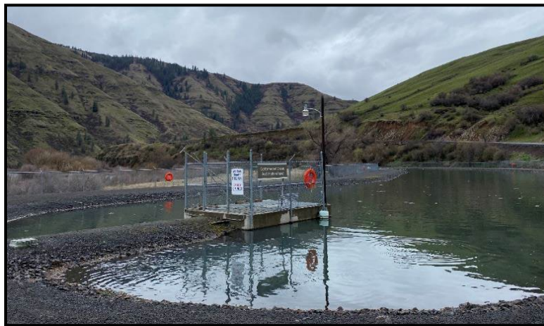
Figure 8. A photograph of the Cottonwood Acclimation Facility.
