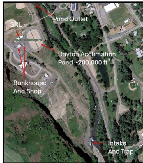
Figure 5. An aerial photograph of the Dayton Acclimation Pond and site-specific structures.
