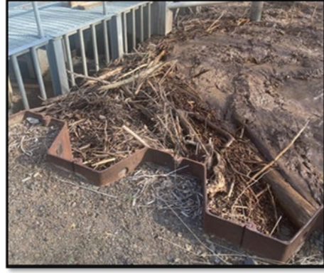
Figure 5. Sedimented raceway following flood event. Figure 6. Clogged Intake Structure.
