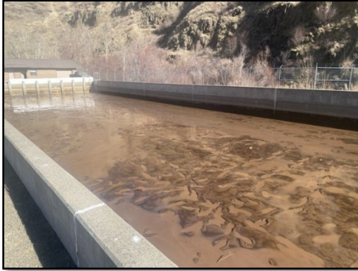
Figure 5. Sedimented raceway following flood event. Figure 6. Clogged Intake Structure.
