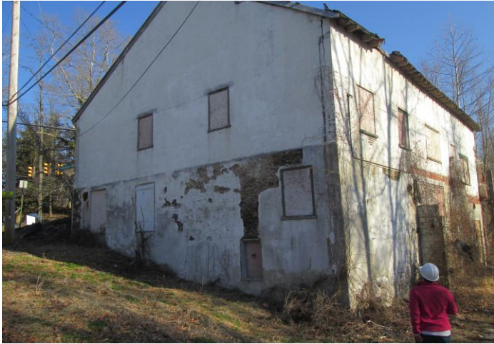
Photo 7 - Southeast corner of structure
