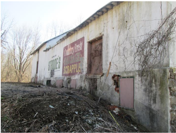
Photo 9 - West side of building
