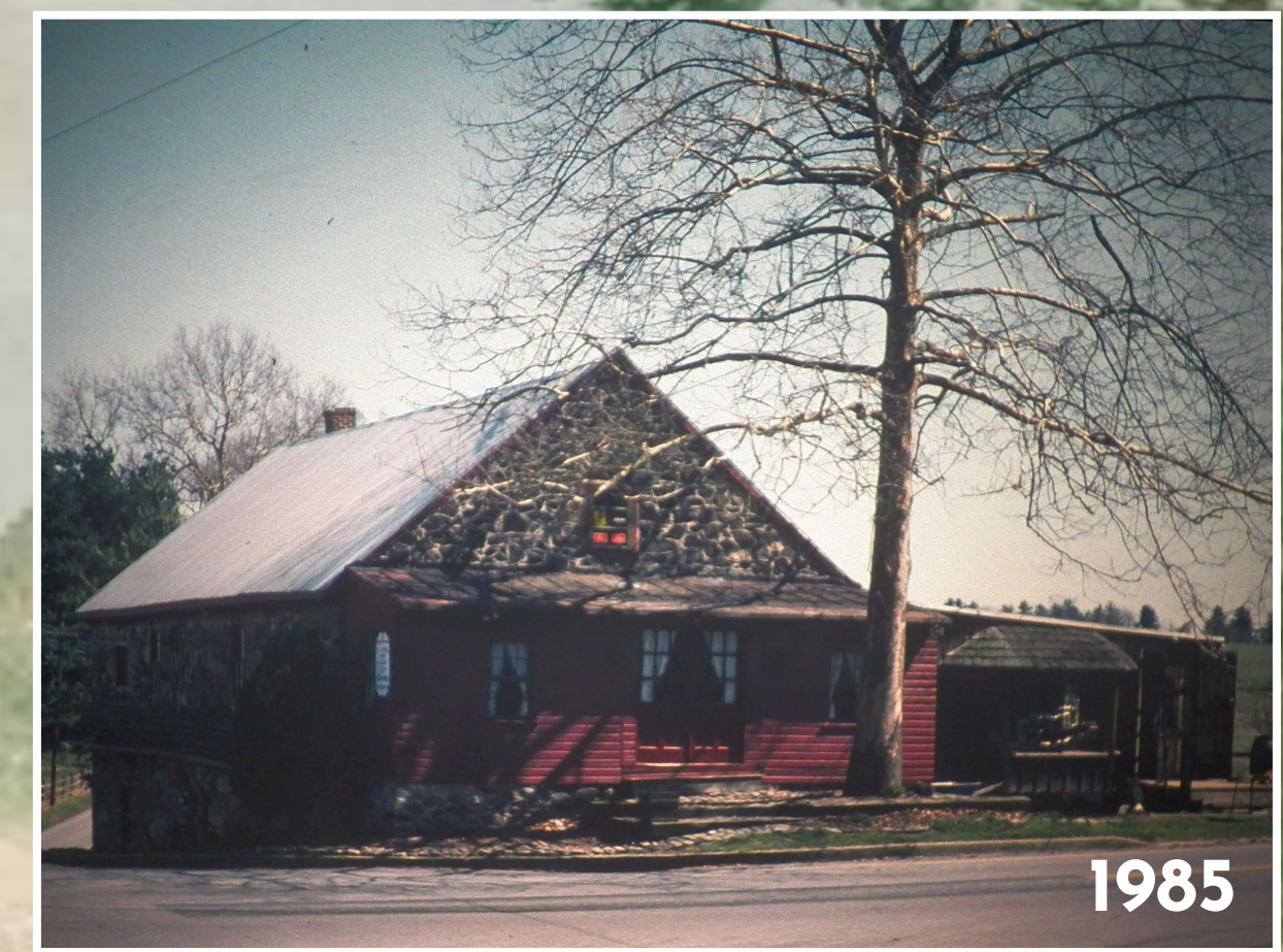
Photograph of Strode's Mill by East Bradford Township, taken in 1985 while under the ownership of Harry J. Waite. Courtesy of East Bradford Township
