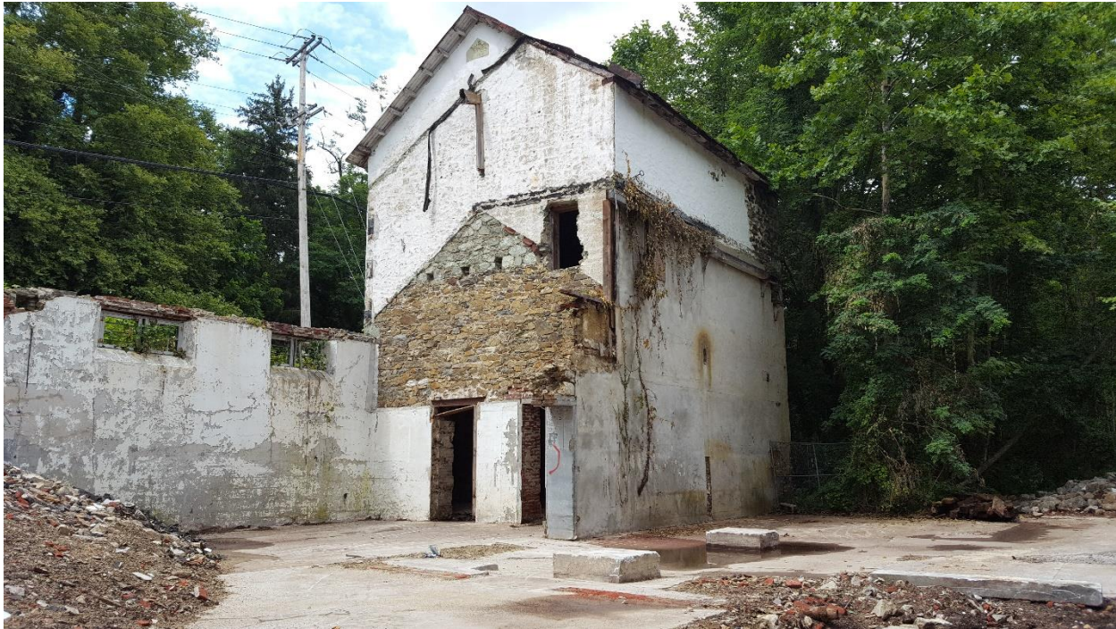
Figure 1-1 Photograph of Project Site, Former Scrapple Factory
