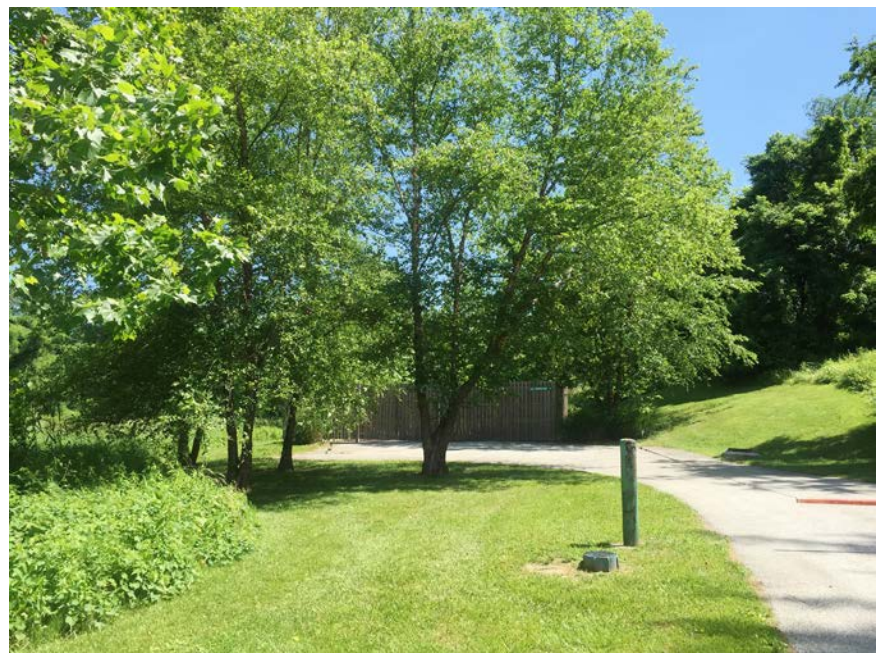
Pump station and potential events parking area
