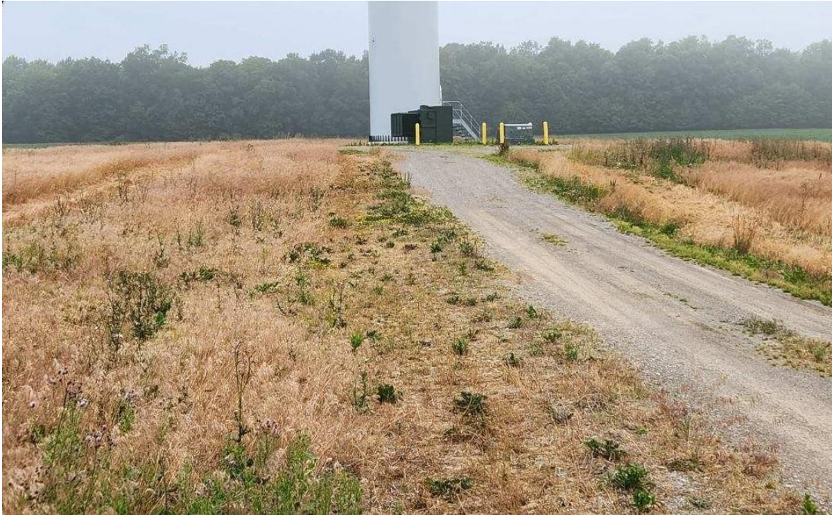
Figure 2. Representative photo of conditions of a 100-meter (328-foot) road and pad plot at the Crescent Wind Project, Hillsdale County, Michigan.
