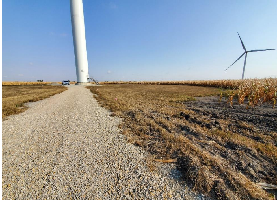
Figure 4. Example of a 40-meter cleared plot at the Green River Wind Farm, Lee and Whiteside counties, Illinois, showing the gravel road and pad associated with a turbine and the mowed area maintained at cleared plots and hybrid plots.
