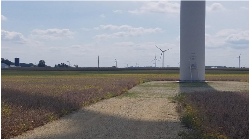
Figure 2. Representative photo of conditions of a 100-meter road and pad plot at the Headwaters Wind Farm, Randolph County, Indiana, from April 1 – July 31, 2022.
