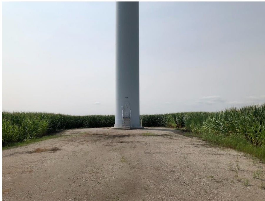
Figure 3. Representative photo of conditions of a 100-meter road and pad plot.
