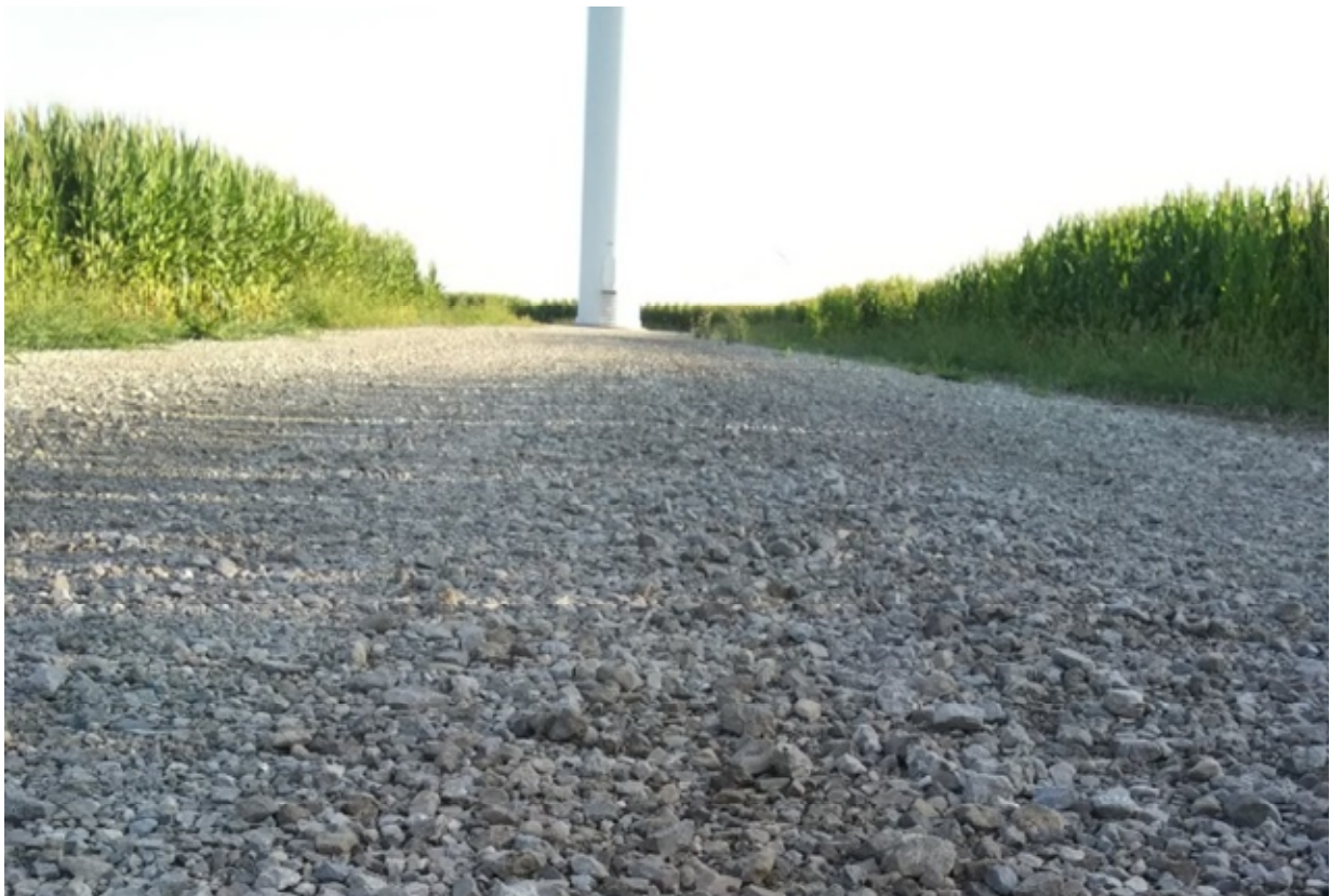
Figure 2. Representative photo of a 100-meter road and pad plot.
