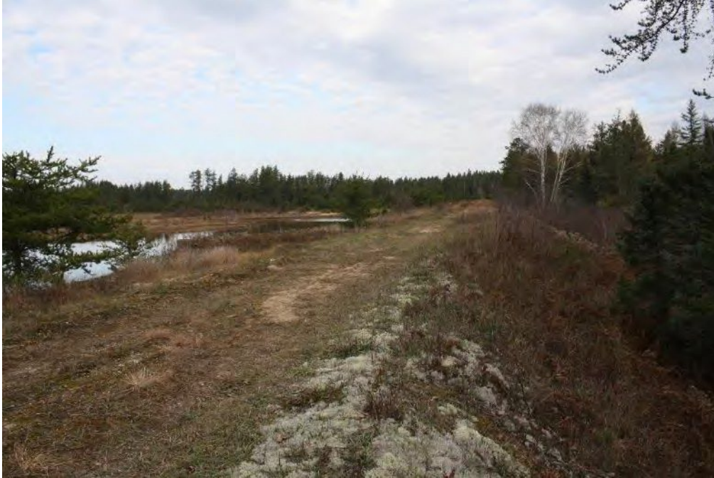
Figure 22 Project Area, Delta Creek Dam, view to the northeast
