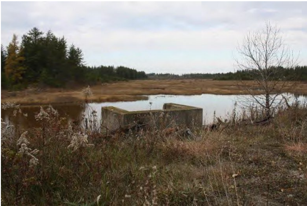
Figure 15 Project Area, west bank of Delta Creek Pool and water control structure, view to the north
