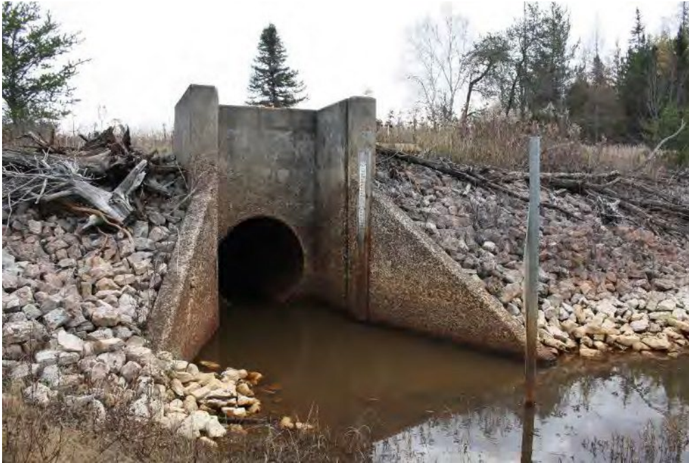
Figure 16 Project Area, water control structure, view to the southeast
