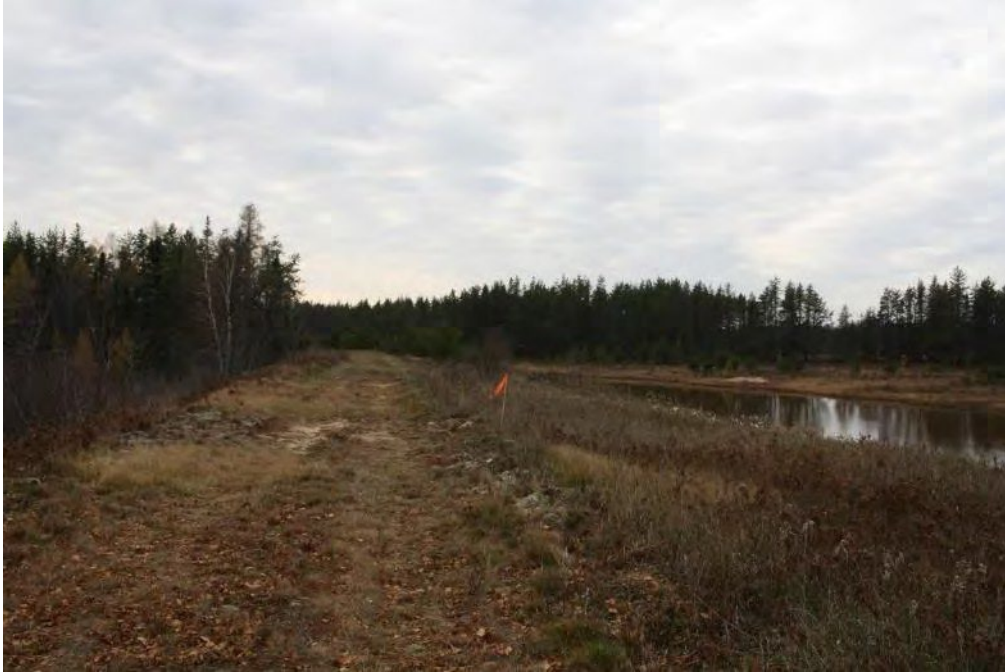
Figure 18 Project Area, Delta Creek Dam, view to the southwest
