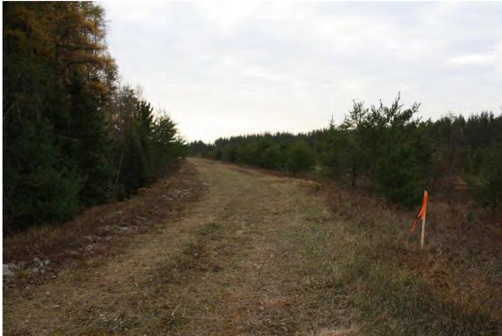
Figure 12 Project Area, Delta Creek Dam, view to the south
