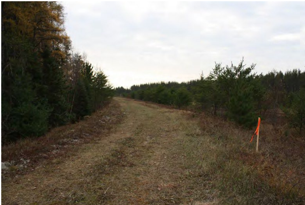
Figure 2 Dam Low Hazard - Delta Creek Pool, view to the south
