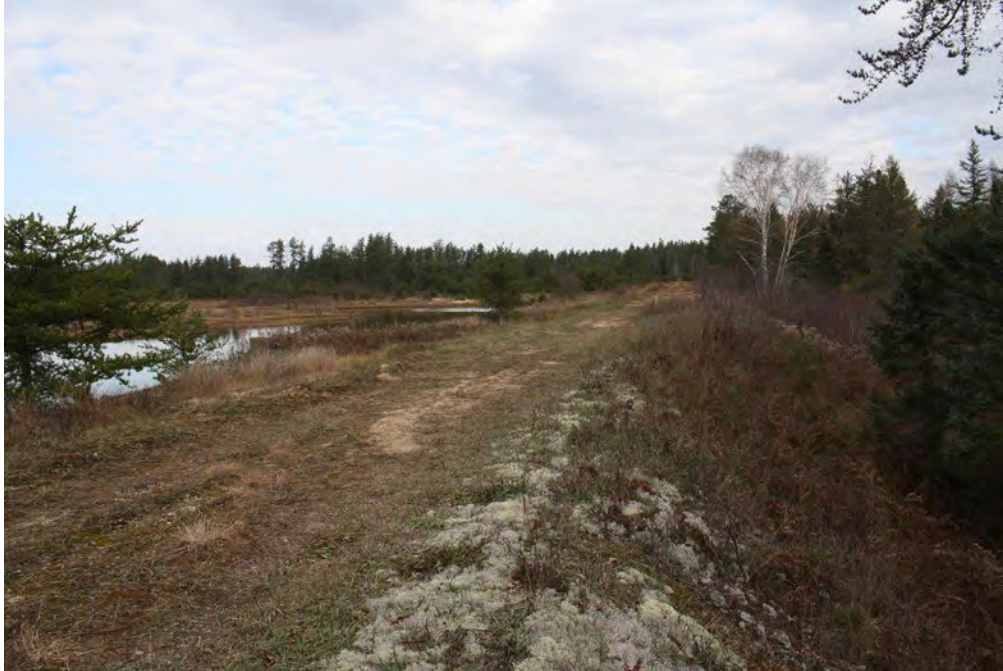
Figure 5. Dam Low Hazard - Delta Creek Pool, view to the northeast
