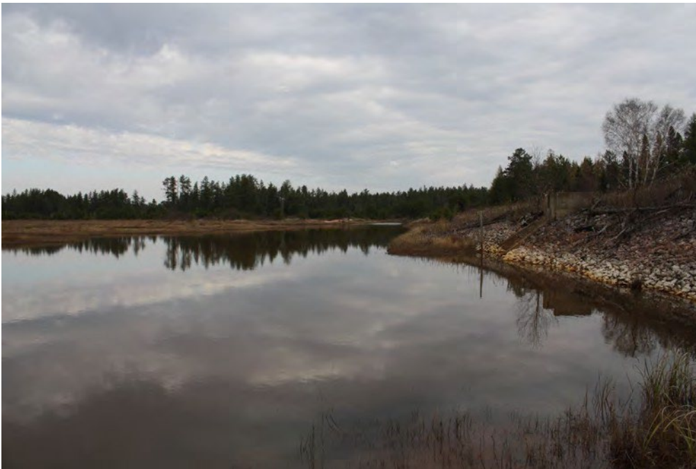
Figure 2. Delta Creek Pool to Delta Creek water control structure, view to the northeast
