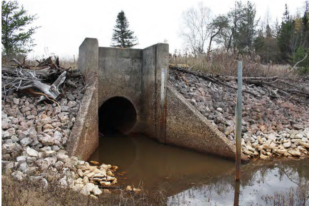
Figure 11 Project Area, water control structure, view to the southeast
