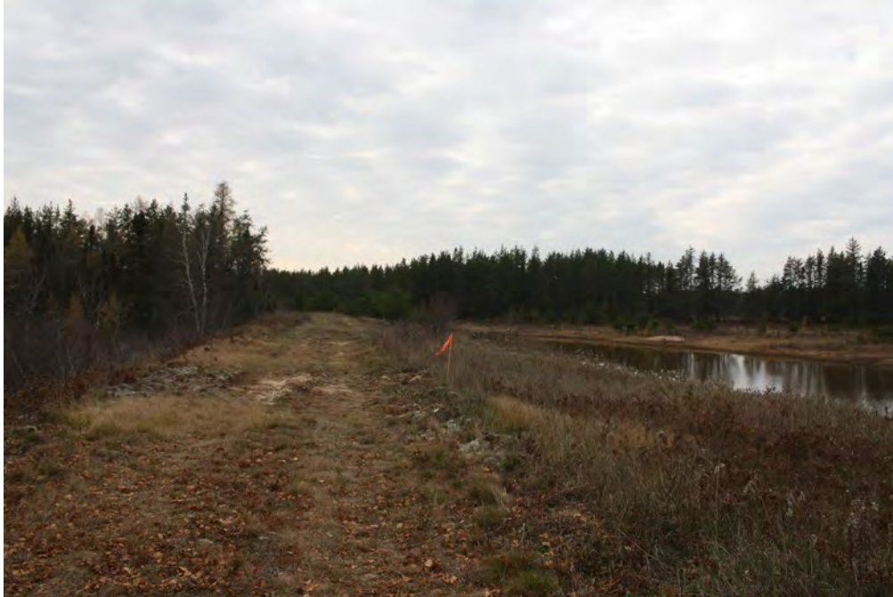
Figure 3 Dam Low Hazard - Delta Creek Pool, view to the southwest
