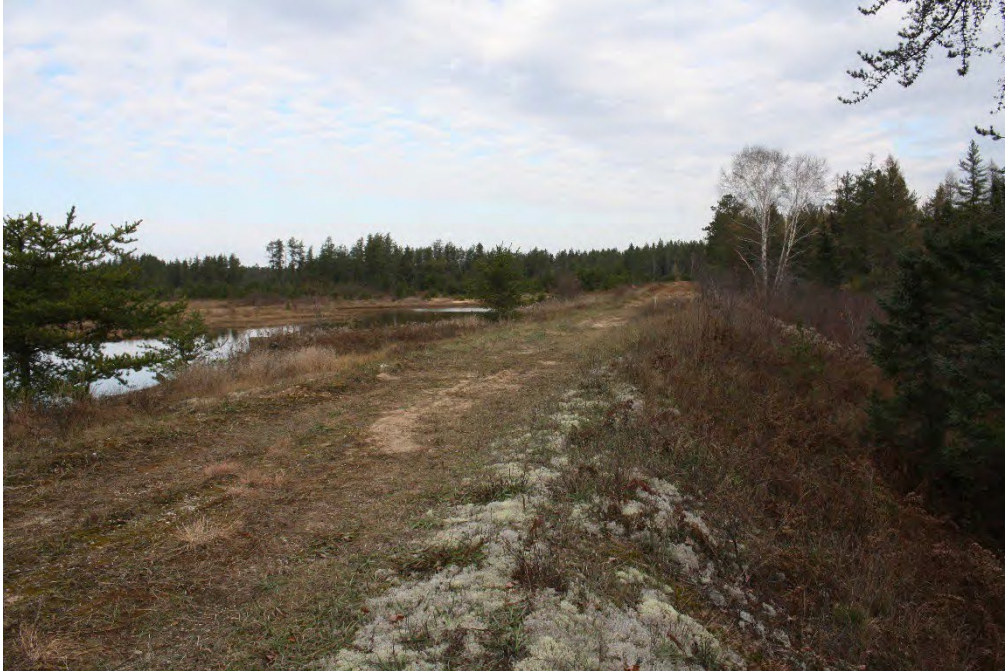
Figure 17 Project Area, Delta Creek Dam, view to the northeast
