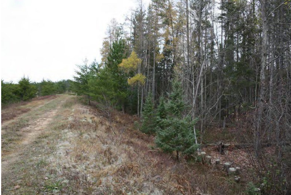
Figure 1 Dam Low Hazard - Delta Creek Pool, view to the north
