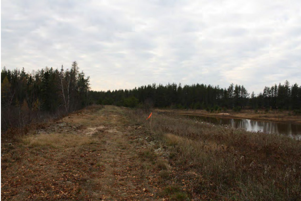
Figure 13 Project Area, Delta Creek Dam, view to the southwest
