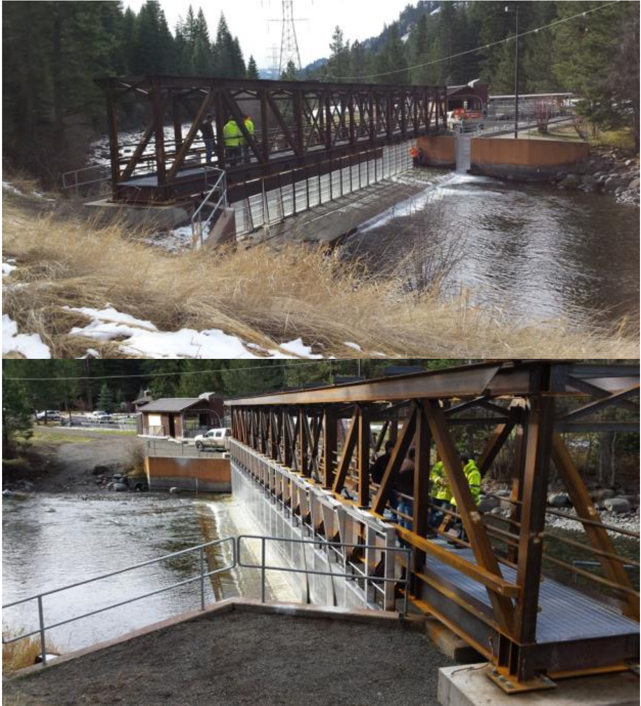
Figure 2. Pictures of the new bridge-style weir installed at the Innaha River acclimation facility and brood collection ponds during October 2015. Weir panels are in the “down” position and pivot from the lower portion of the bridge to operate. Photos by USFWS – Lower Snake River Compensation Plan Office.
