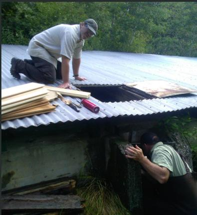
Dam board replacement of both cold spring boxes to improve and conserve cold-water transfer to the wet labs.
