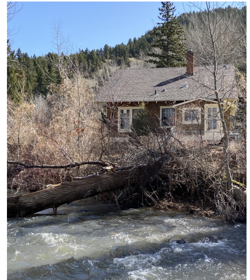
Quarters 2, southwest corner of the structure.
