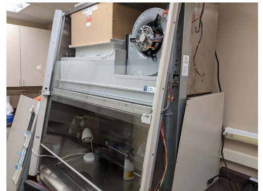
Virology hood repair. Photo: USFWS/Rick Cordes
