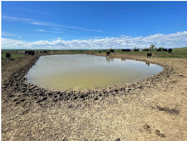
Figure 21. South Stock Dam
