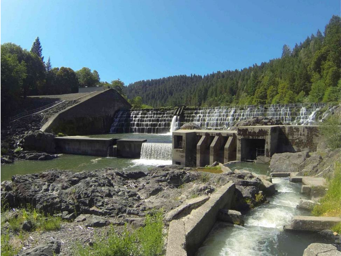
Figure 5. Cape Horn Dam on the Eel River. The dam and fish ladder restricts passage of Pacific Lamprey to upstream reaches and is being used to study lamprey passage capabilities and test lamprey specific passage facilities. In 2016, a new lamprey passage and minoring system was installed, with 11,506 lampreys counted passing in 2017.
