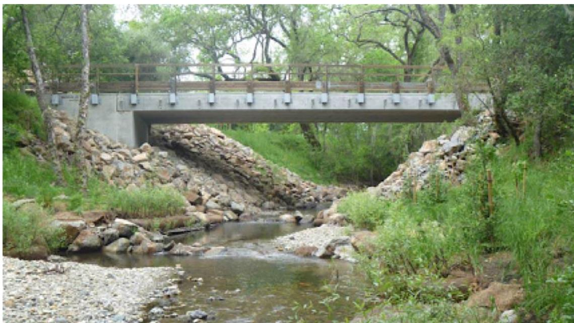
Figure 5. The Greenwood Road culvert was initially identified as a total barrier to Pacific Lamprey on mainstem Napa River, although resident brook lamprey occur upstream, indicating habitat suitability. The culvert was removed in 2015 by NRRCD and replaced by a bridge, opening access to 2.75 mi of habitat below Kimball Canyon Dam.
