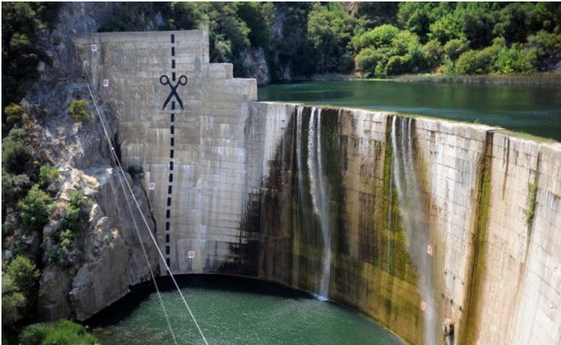
Figure 4. Matilija Dam is the current extent of anadromy on Matilija Creek and is located 16 miles upstream from the Ventura River estuary. This 168 ft tall dam is being considered for removal and would increase the extent of anadromy for Pacific Lamprey and Steelhead, as well as provide more natural streamflow regime. Photo taken by Anthony Plascencia of the Ventura County Star.
