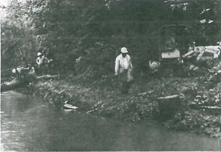
Figure 15. Hand labor crew hooking cable to log to be pulled from stream by small crawler tractor with winch. Only a narrow work zone along the stream was disturbed because of the small equipment. Note stump left in place to stabilize bank.
