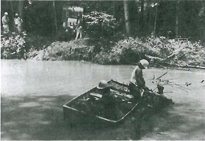
Figure 14. Hand labor crew in boat hooking cable to log. The small crawler tractor with winch will pull the log from the stream. Small equipment can be carefully maneuvered through the floodplain forest causing little damage.
