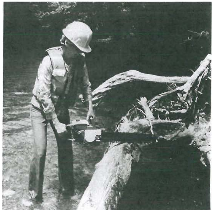
Figure 13. Chainsaw being used to cut log so that it can be pulled with small hand winch and repositioned along stream bank.
