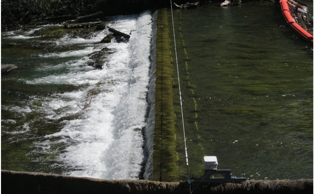
Figure 4. Newly designed flat-plate antenna installed on the upper spillway on September 3, 2014.
