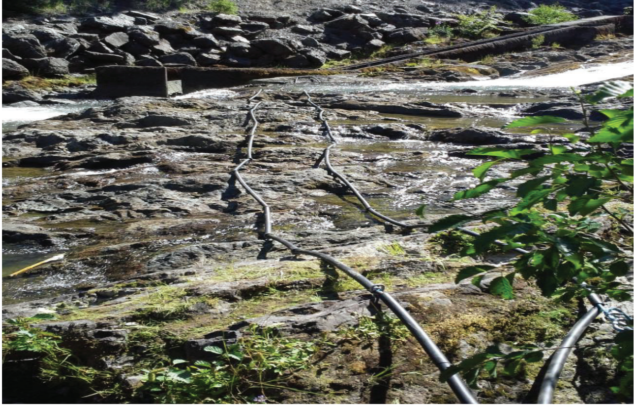
Figure 2. Reinstalled "beaver resistant" lower spillway antenna (July 9, 2014)
