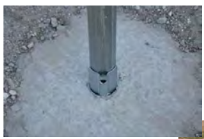
Flexible/Bending Sign Support
